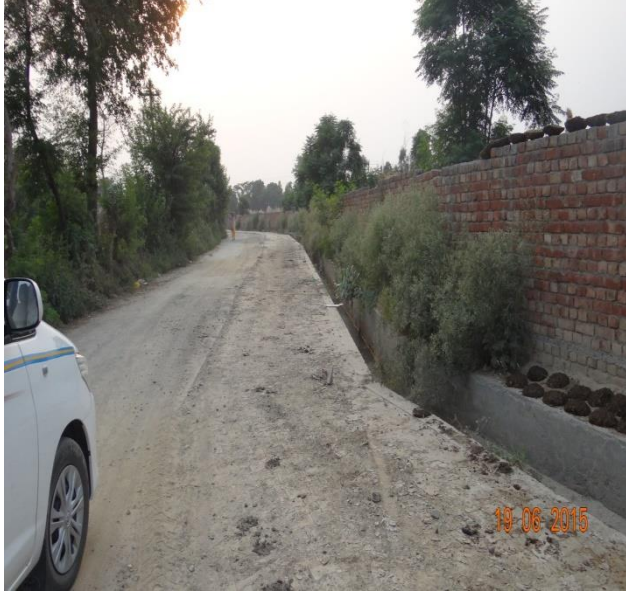
CONSTRUCTION OF INTERLOCKING PATH WITHIN THE VILLAGE
