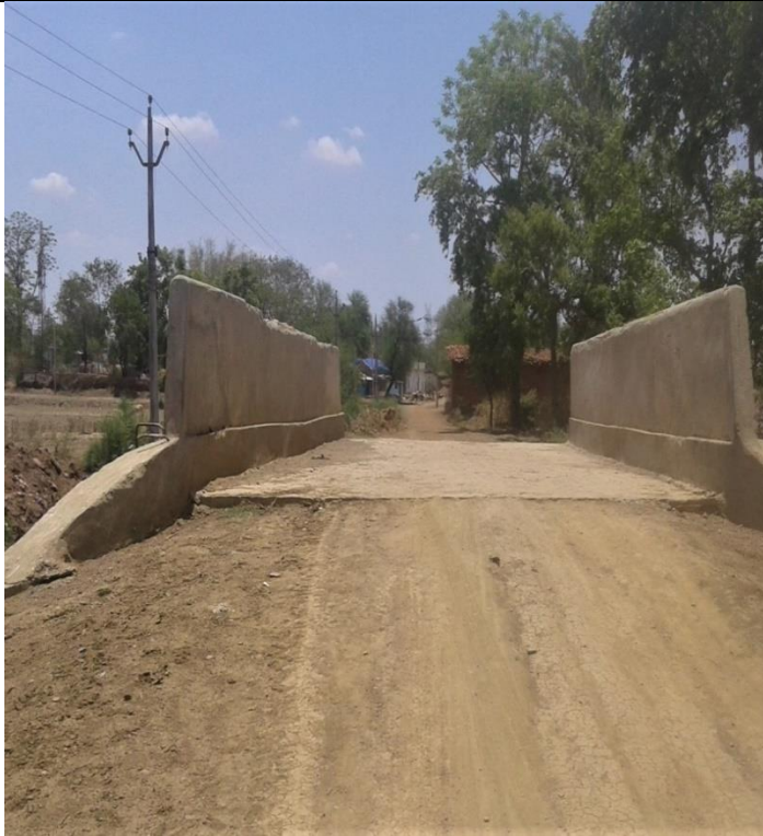
CONSTRUCTION OF RCC BOX CULVERT AT VILL - TAGA
