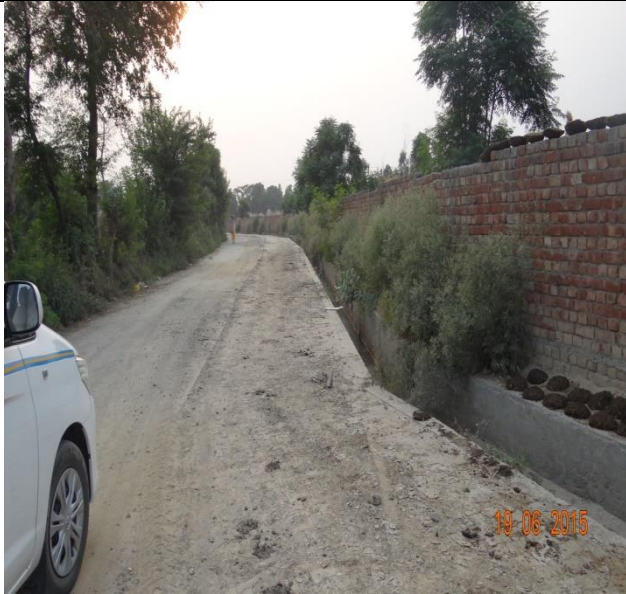
CONSTRUCTION OF INTERLOCKING PATH WITHIN THE VILLAGE
