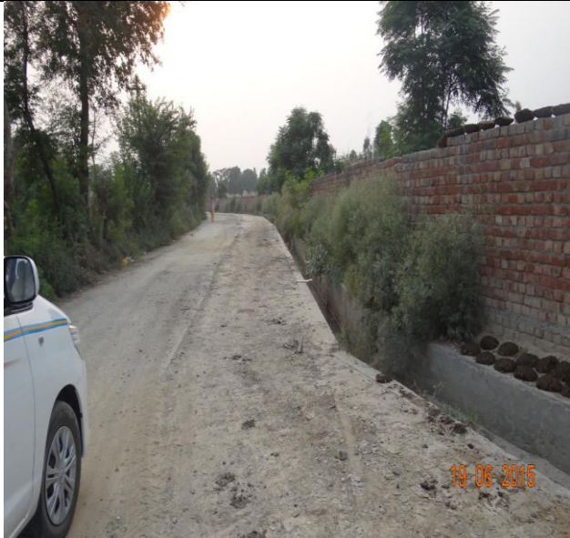
CONSTRUCTION OF INTERLOCKING PATH WITHIN THE VILLAGE
