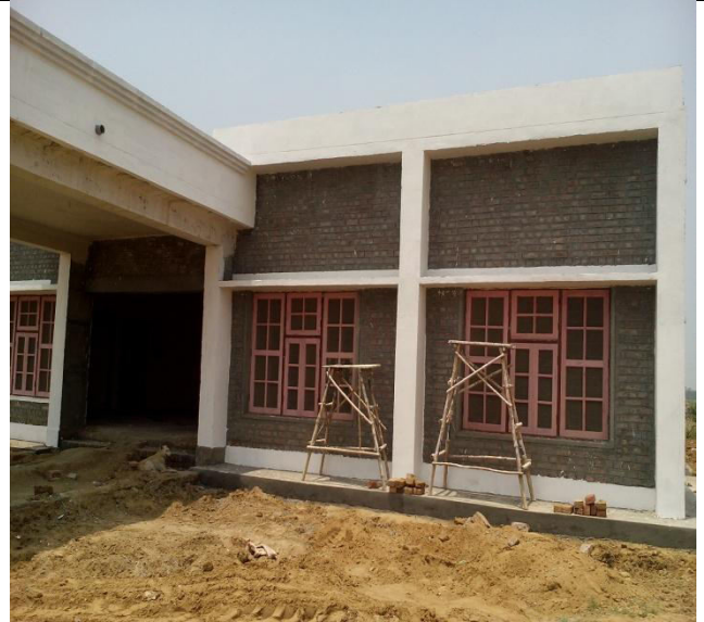
CONSTRUCTION OF COMMUNITY CENTRE
