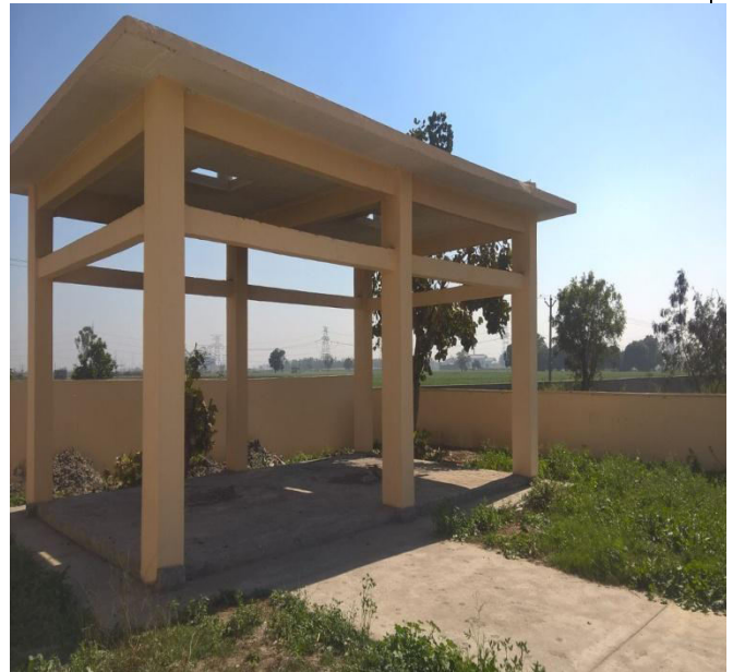
CONSTRUCTION OF SHED AT SHAMSHAN GHAT
