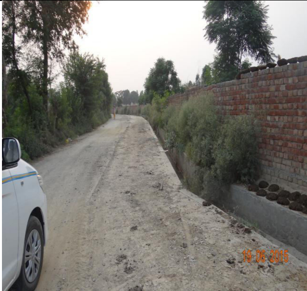
CONSTRUCTION OF INTERLOCKING PATH WITHIN THE VILLAGE
