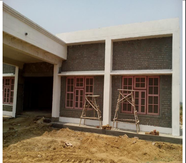
CONSTRUCTION OF COMMUNITY CENTRE
