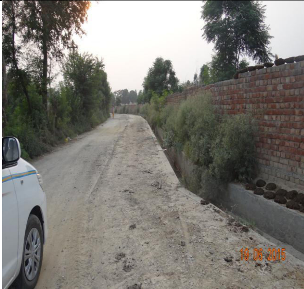
CONSTRUCTION OF INTERLOCKING PATH WITHIN THE VILLAGE
