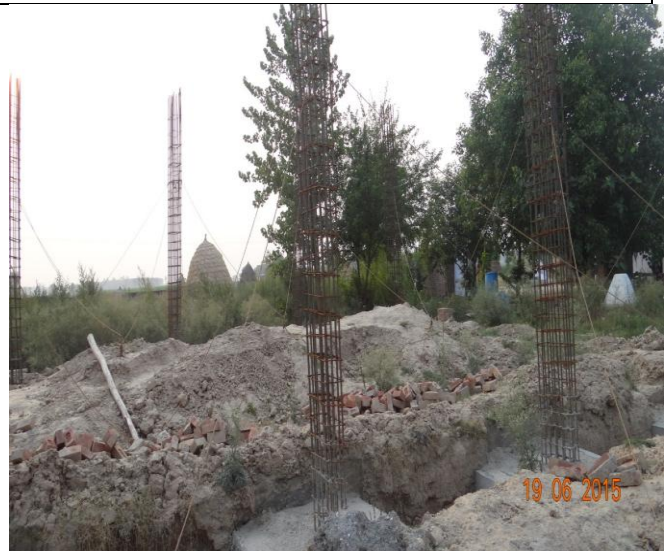
CONSTRUCTION OF COMMUNITY CENTRE
