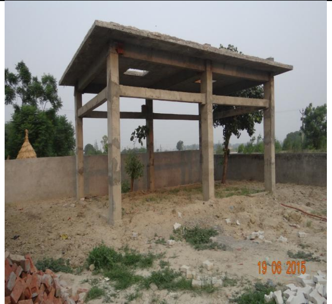
CONSTRUCTION OF SHAMSHAN SHED
