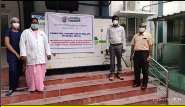
DG Set for Govt. Hospital, Kallakurichi, Tamil Nadu
