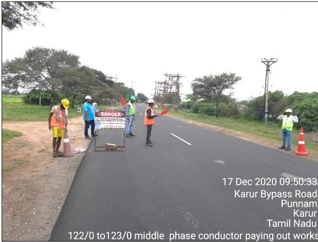
Traffic Management during stringing activity over road & ensuring availability of First Aid Kit
