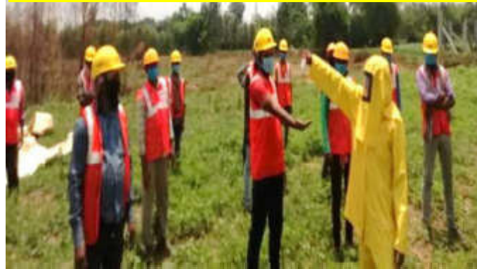
LOC. No. 75/0 for Moktarul Islam(Tower Erection work)
