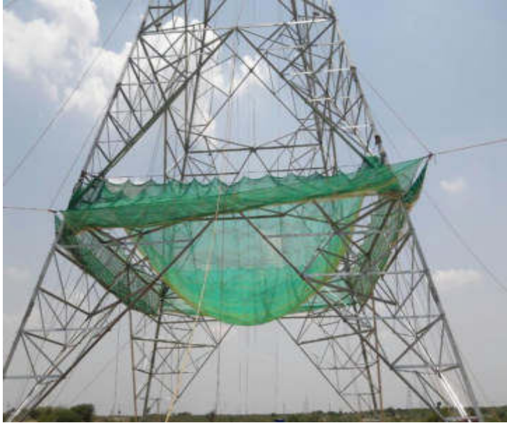
Usage of Safety Nets during tower Erection work (Pavagada- Devanahalli line)
