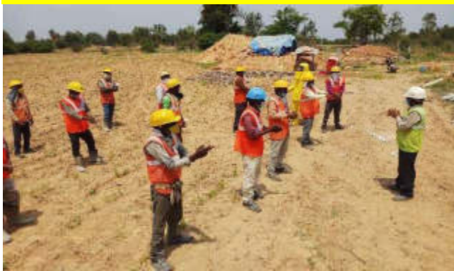
LOC. No. 86/0 for SSV Gang (Foundation work)
