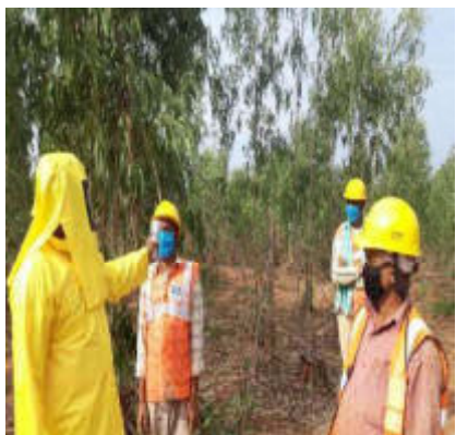
Moktarul Gang at Loc. 75/0 (Tower Erection)
