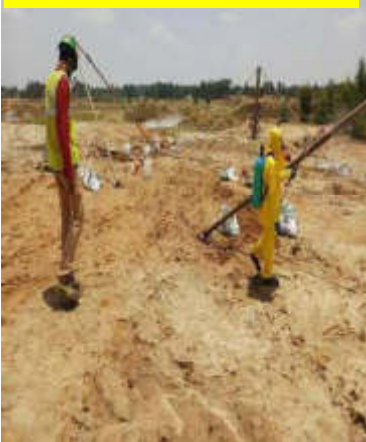
At loc no. 88/0 for SV const. (Foundation)
