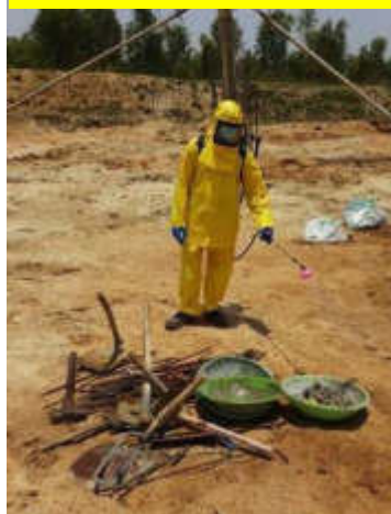
At SV const. (Foundation)
