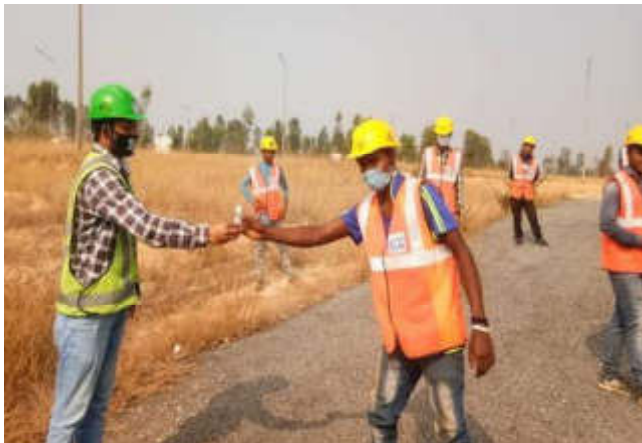
Loc No 124 Moktarul Islam Gang for Stringing work
