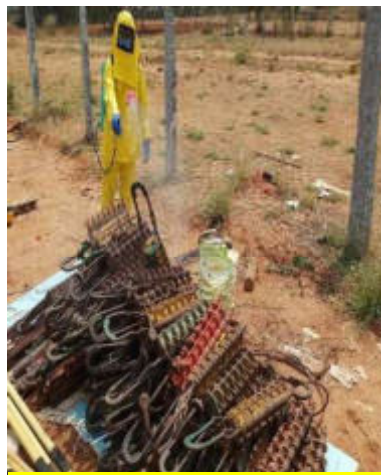
At K. Kumar gang (Stringing)
