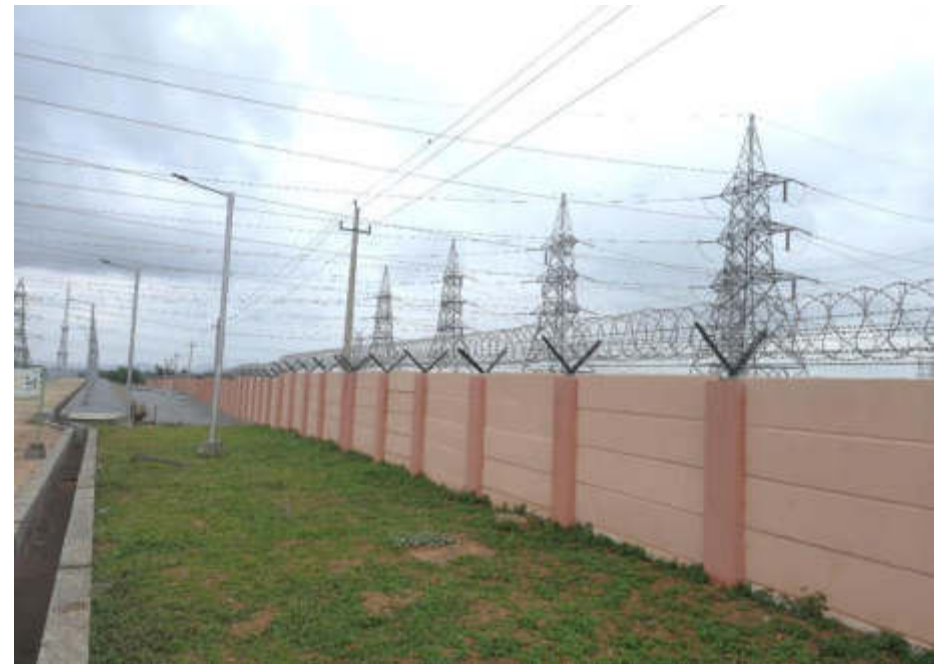
Security fence at Pavagada Substation
