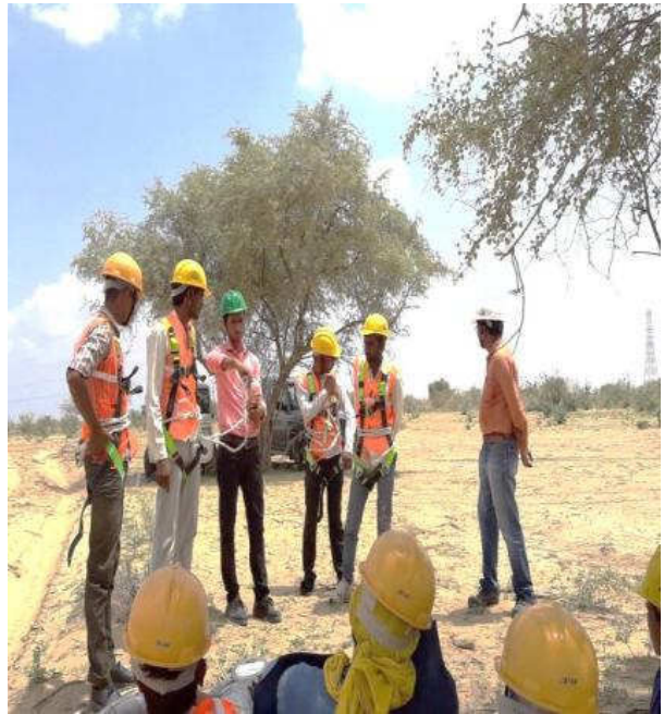
Safety Training at Work sites (Bhadla-Bikaner Line)
