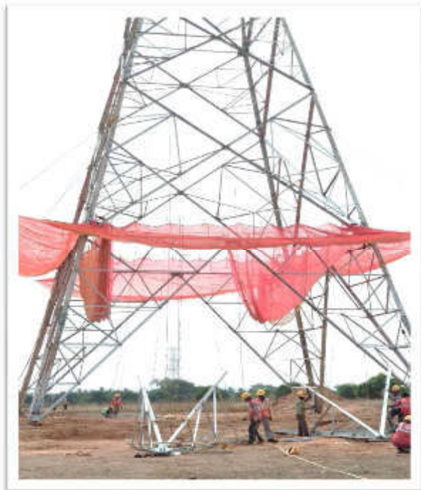
Usage of Safety Nets during Tower Erection works (Pavagada - Devanahalli Line)
