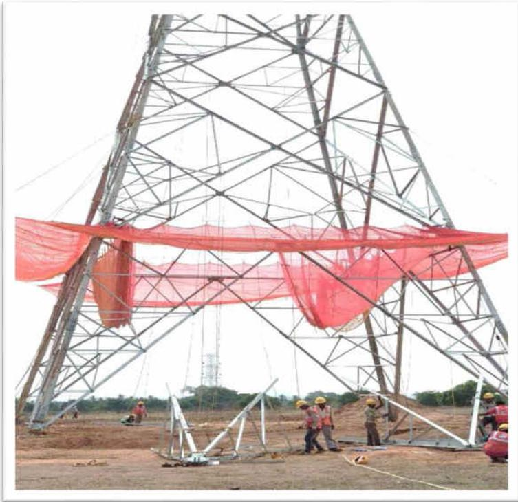
Usage of Safety Nets during Tower Erection works Pavagada Devanahalli Line, Location- AP 23/0 (March'18)
