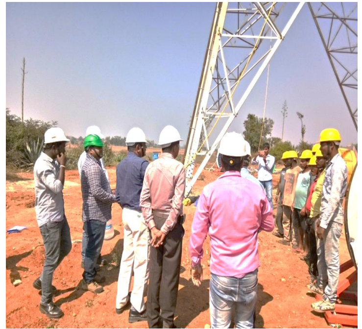
Tower Location-AP-97/0 Hiriyur –Mysore Line, Tower No. Date: 27.12.14
