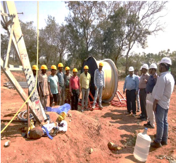
Tower Location- AP-97/0 Hiriyur –Mysore Line, Tower no. Date: 27.12.17
