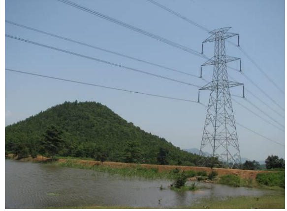
Plate - 2: Power Grid Line along forest area
