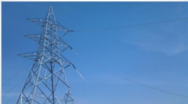
Conductor Rough Sag in progress
