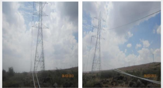
Conductor Payout through Suspension Towers
