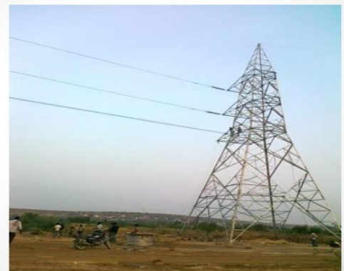
Conductor Stringing Completed
