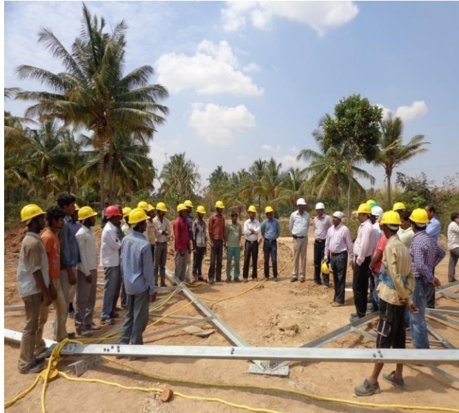
Safety meetings before commencement of construction work
