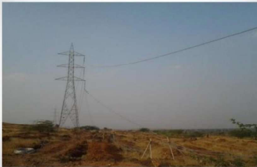
Conductor Payout for each Phase
