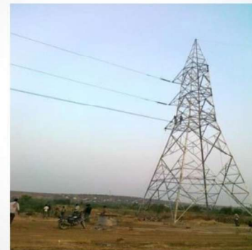
Conductor Stringing Completed
