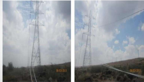
Conductor Payout through Suspension Towers
