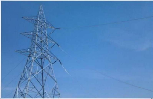
Conductor Rough Sag in progress
