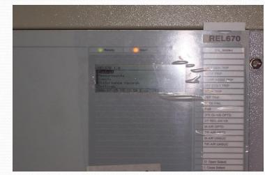
SIMILARLY, BAY CONTROL UNIT WHICH IS BEING USED FOR ANALOG AND DIGITAL DATA ACQUISITION AND BAY EQUIPMENT CONTROL FUNCTIONS HAS ALSO AUTO VOLTAGE CHECK SYNCHRONISING FUNCTIONS AND AUTO RECLOSURE FUNCTIONS.
