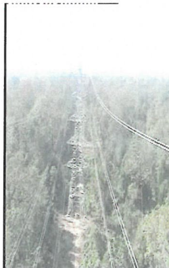
Multi Circuit Tower Erection Using Existing Corridor in Jaldapara Sanctuary
