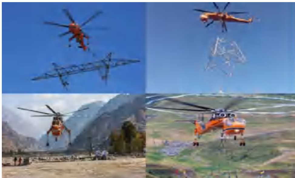
Figure 24: Using Helicopter for Tower Erection in Himalayan Valley in India
